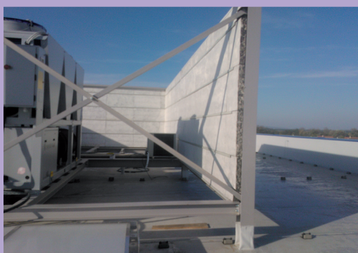
Protihluková stena Noise barrier
