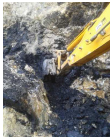
Fig. 2.3. Finishing of cleaning works from the crevasses of quarry
