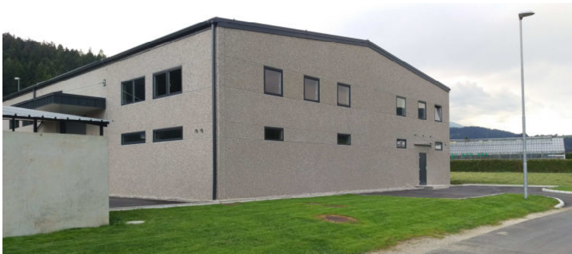
Fig. 2. Demonstration plant for soil washing technology.
