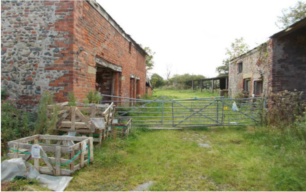
Fig. 1. Redundant farm buildings scheduled for residential redevelopment.
