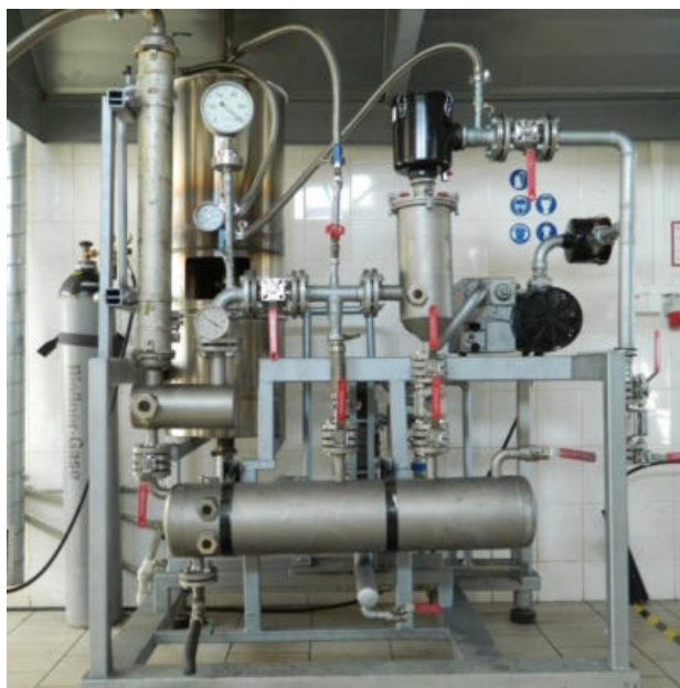
Fig. 3. Condensation unit of semi-pilot testing unit.
