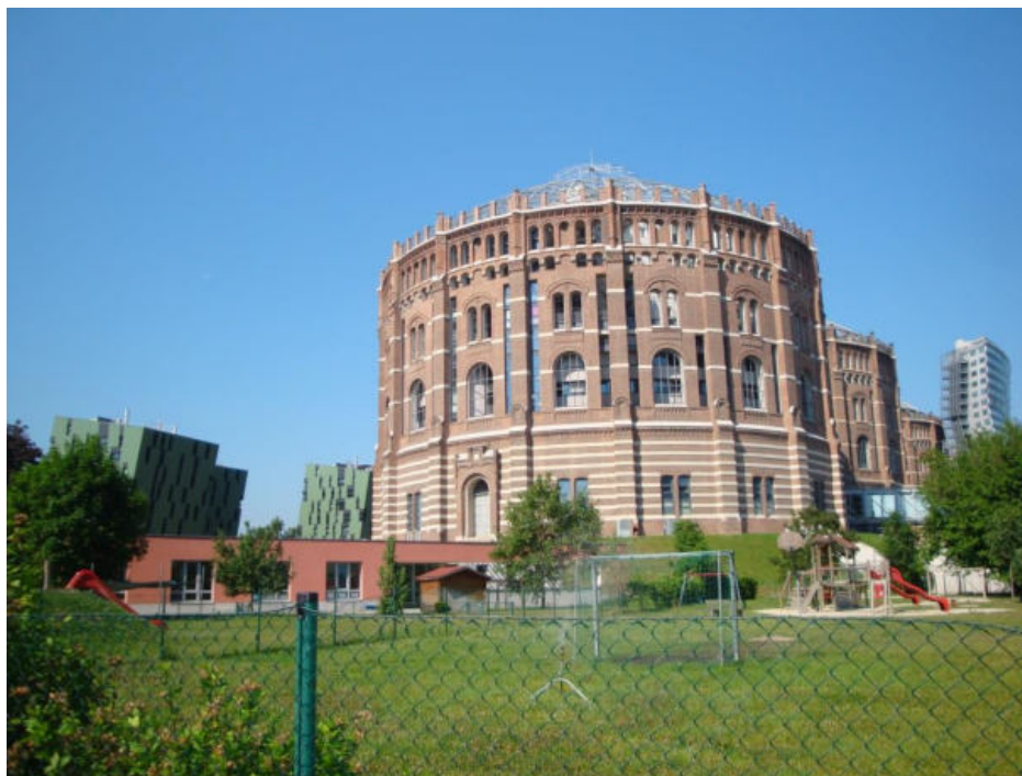
Fig. 3. “Gasworks Simmering” after rehabilitation - (source: Environment Agency Austria)
