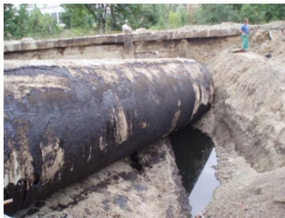
Fig. 2. Removal of the underground storage tanks at Bratislava-Rača
